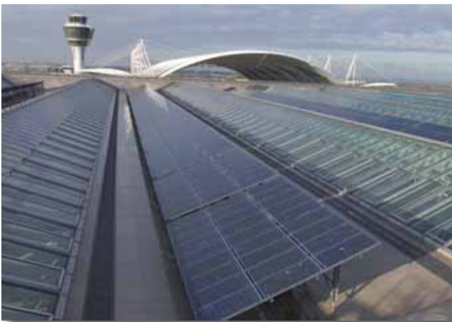
Silicon photovoltaic systems engineered for low maintenance and long-term environmental exposure are being used increasingly on commercial buildings worldwide. This 457-kW array was installed on the roof of the Lufthansa terminal at Munich Airport in 2002. (photo: BP p.l.c.)
